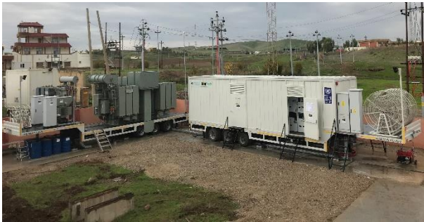
MOBILE SUBSTATION-ERBIL,IRAQ
