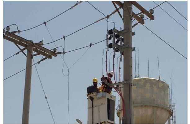
11kV OHL CONNECTION BALAD AB/IRAQ
