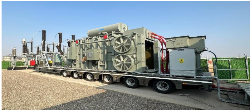
132/33kV 63 MVA MOBILE SUBSTATION BAGHDAD-IRAQ
