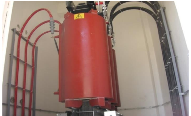
ADANA TUYAP FAIR AREA 4*33kV/1600kVA DRY TYPE SS
