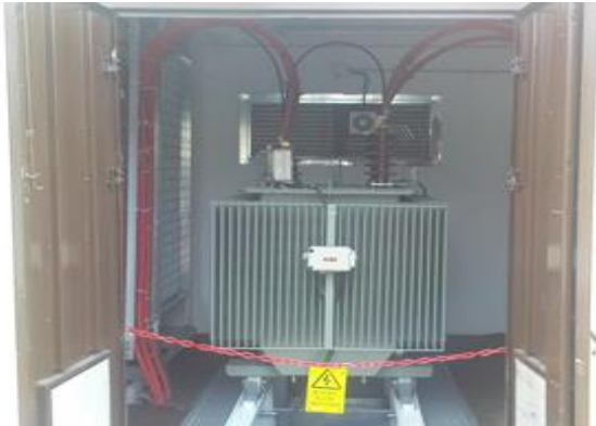
POWER TRANSFORMER INSTALLATION 33/6,3kV 1,6 MVA USA ASF ANKARA
